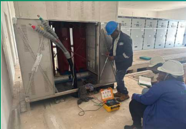
Fig. 4 100MW Solar Project Switchgear room expansion electrical test ongoing on switchgears
