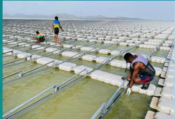
Fig. 3 completed installation of 5MW mounting structures for the 20MW floating solar project
