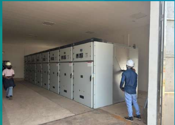
Fig. 4 100MW Solar Project Switchgear room expansion electrical test ongoing on switchgears
